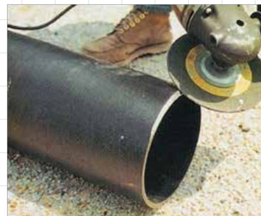
Fig. 5.11.1: Chamfering of DI Pipe Cut Ends
